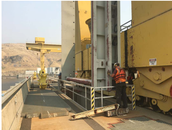
Instrumented ASFM frame being lowered into intake slot.
